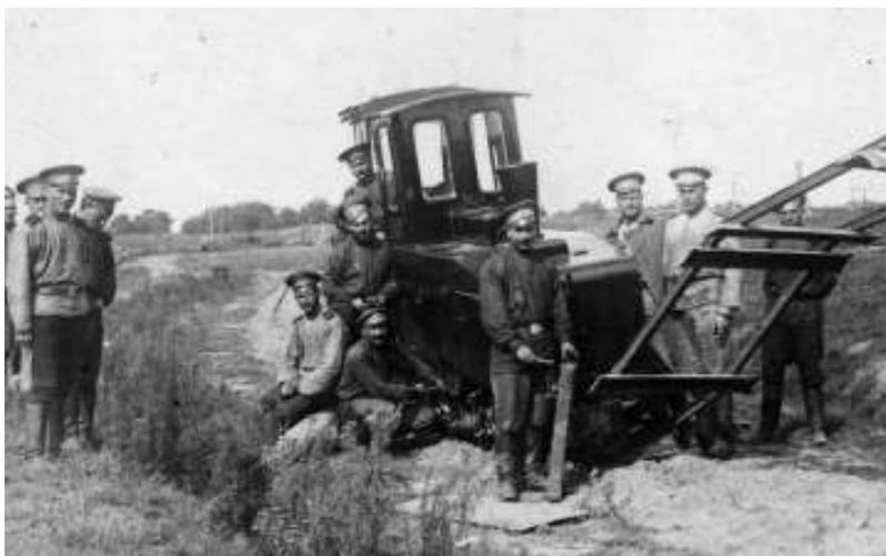
Derailment of Deutz twin locomotives on light portable tracks during trials in the Russian Army, 1910
